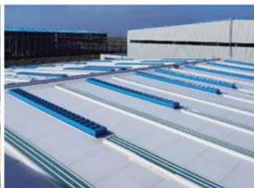
铺设TPO防水卷材
